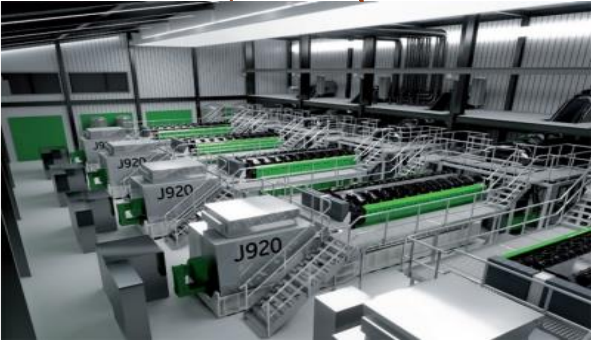
J920 9.5 MW gas engine, developed for on-site power and CHP
